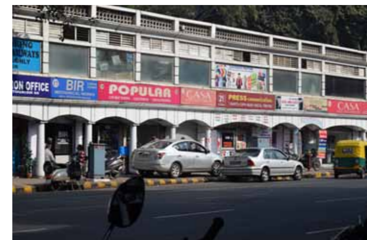
Parking on footpath at Super Bazaar leading to encroachment
