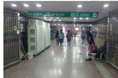
Well maintained grade separated subways on outer circle
