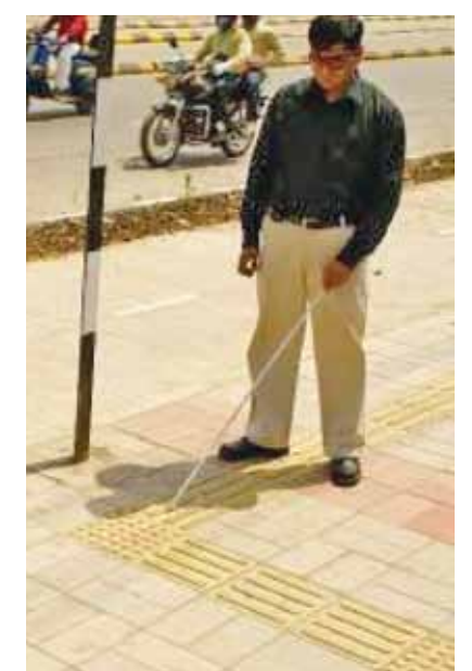
Tactile Paving on Footpath
