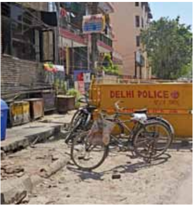
Encroachment on Pilot Stretch
