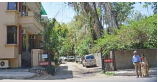
No Provision for Pedestrians/Cyclists
