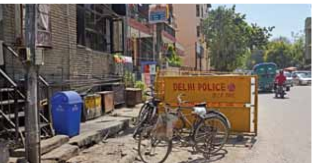
Lack of Maintenance – Footpath
