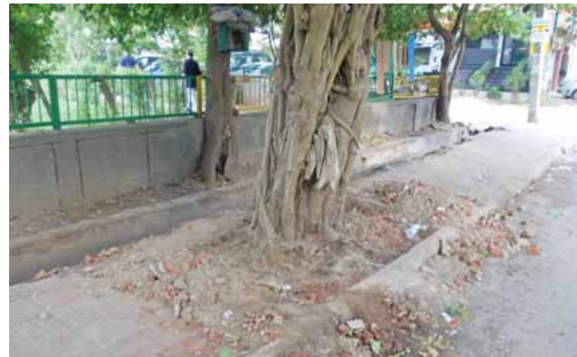
Tree without Grating at Base
