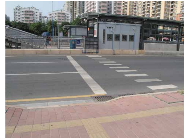
Absence of designated space for the pedestrian and the physically disabled
