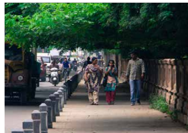
Bollards segregating the pedestrian space from the carriageway
