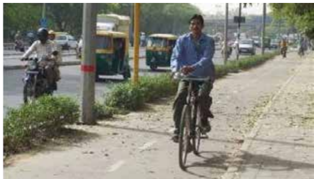
Cycle Track and Carriageway separated by Kerb Stones
