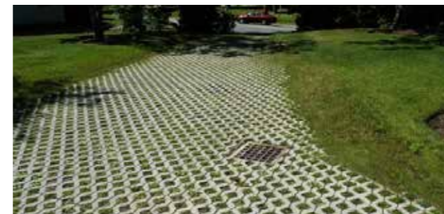
Honeycomb Pavers allow water permeation
