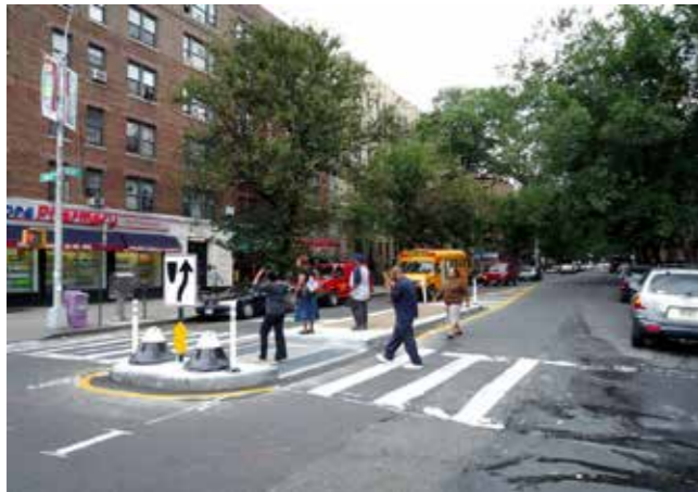
Mid Block Crossing with a Pedestrian Refuge
