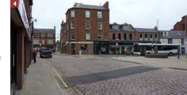
4 Cobble pavement along the pedestrian crossing
