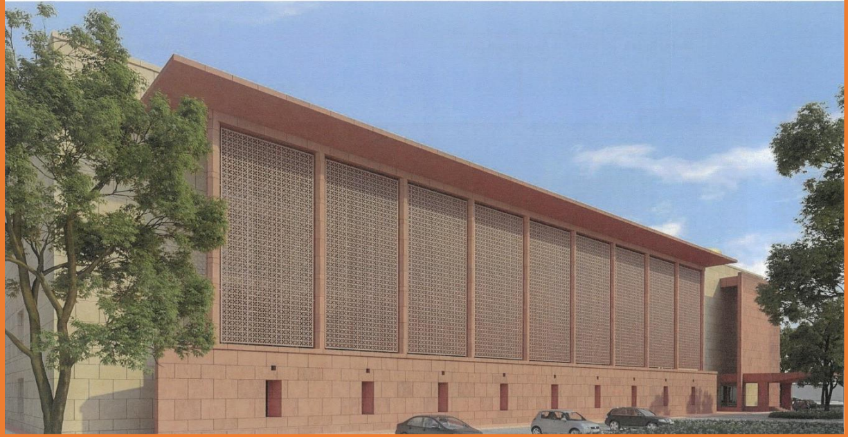
Building Exterior Views
